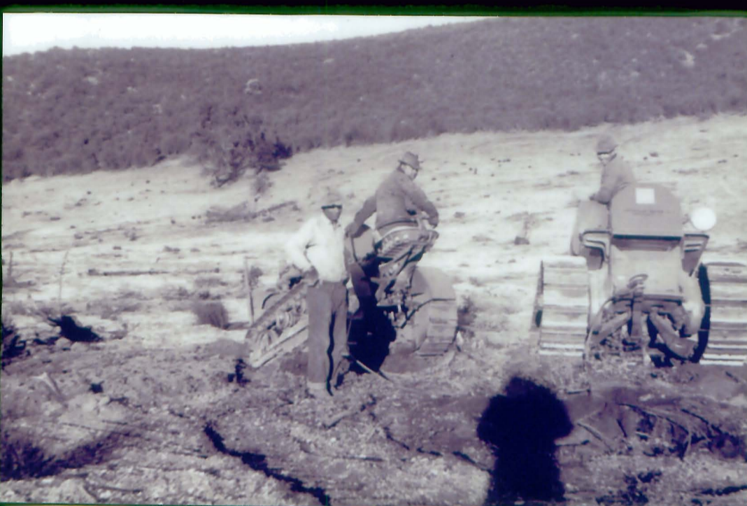
Mervyn, Warren, and a Avila Clearing Stumps
