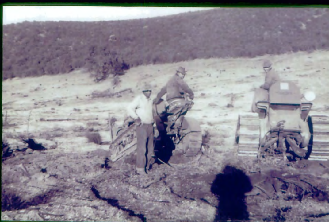
Mervyn, Warren, and a Avila Clearing Stumps
