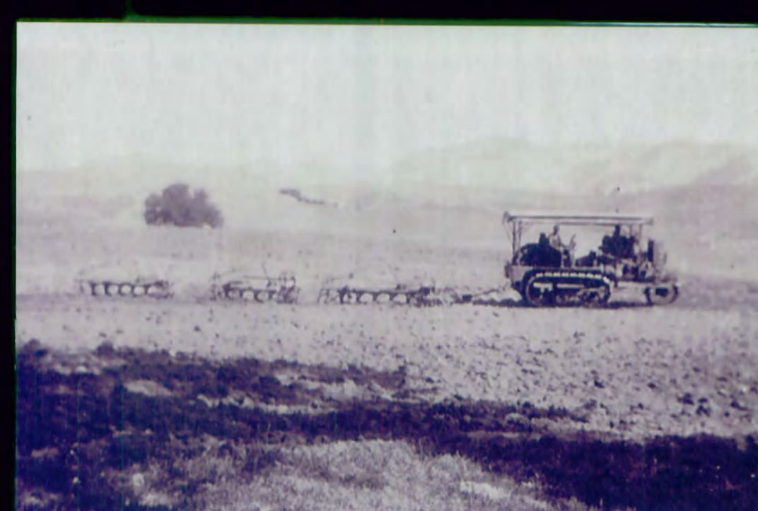
Working Ground in Kirk Canyon
