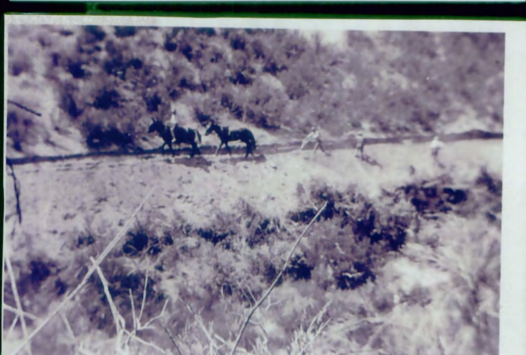
Building a Road to Robinson Canyon Canyon
